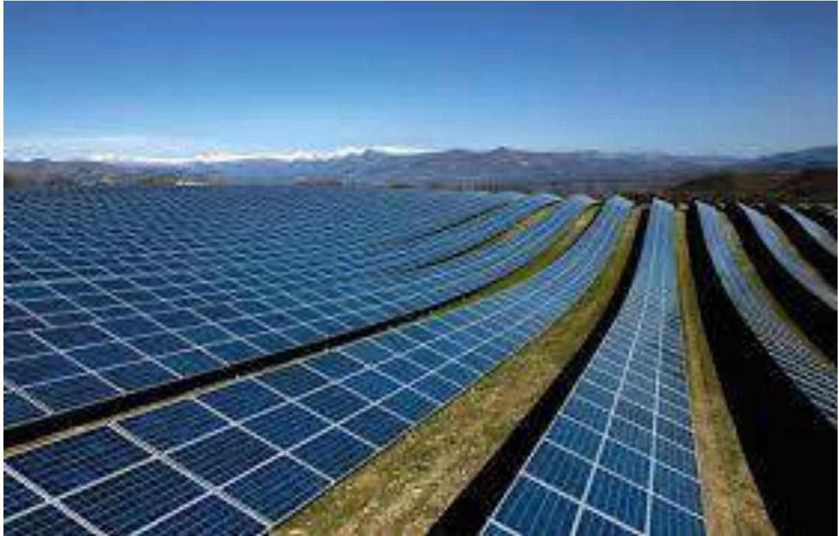
Figure 6.3: Rewa solar power project
